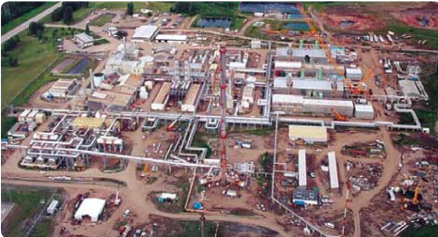
Spectra Energy's Fort Nelson Gas-Processing Plant, northeastern British Columbia, Canada.
