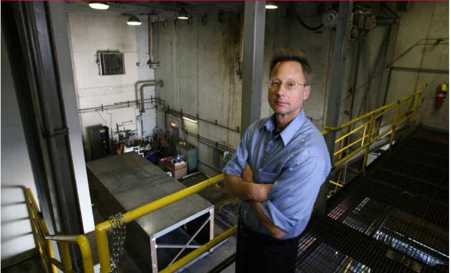
The EERC is modifying the existing “Slurry” Building to be able to accommodate a larger fuel production system to produce liquid jet fuels for testing by the U.S. Air Force. EERC Senior Research Manager Ted Aulich stands on a walkway in the facility, which will soon be modified to house the fuel production system. Aulich is the project manager for the fuel production project.
