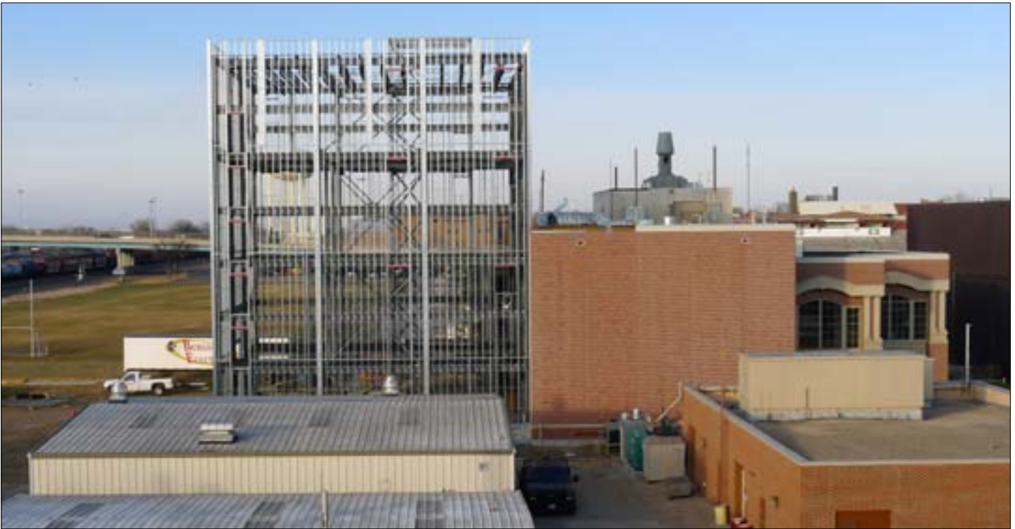
The Fuels of the Future addition to the NCHT building is progressing rapidly, with the steel frame of the high-bay area nearly complete. Tom Erickson, Associate Director for Business and Operations, says the addition should be enclosed by early January and completed in the summer of 2012.
