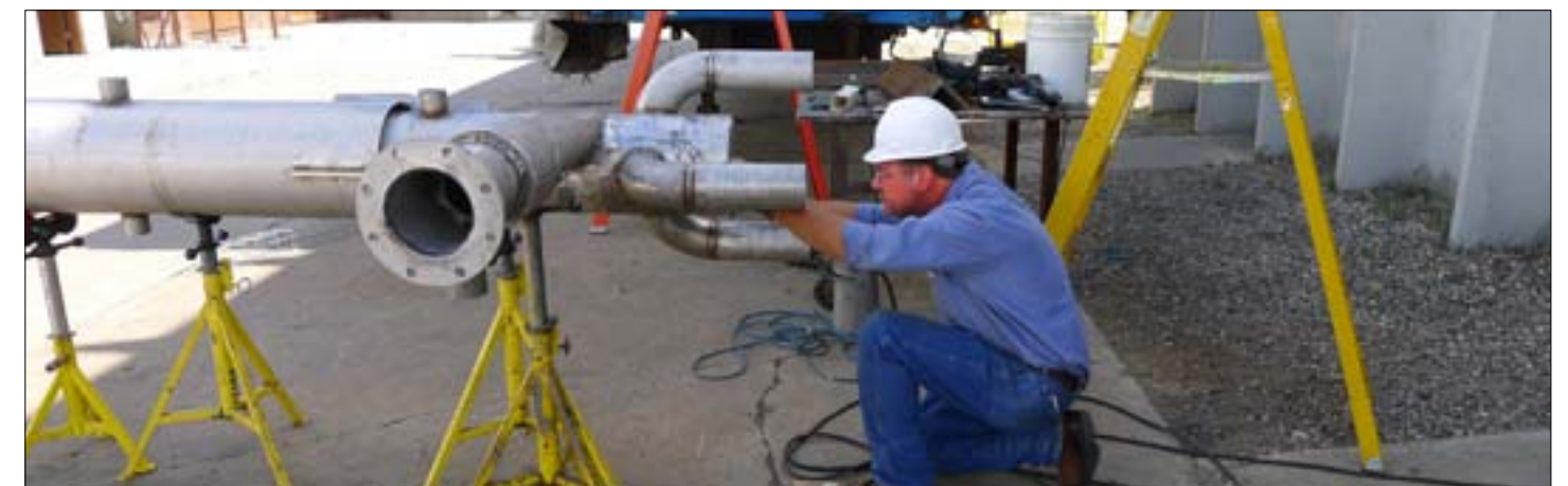
Todd Deibert constructs the flare for the biomass gasification system.
