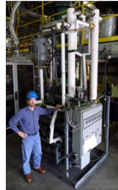
Josh Strege stands by the FT reactor.
