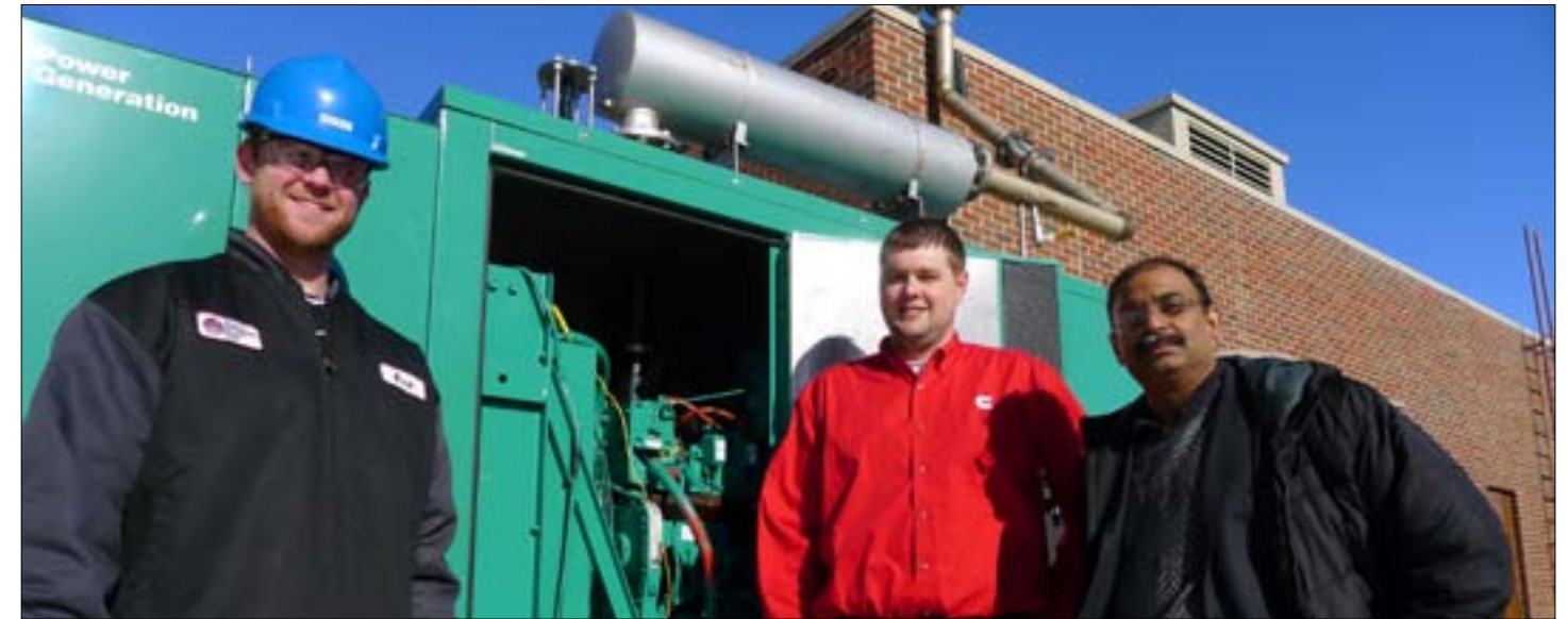
Erik Moe, Research Engineer, EERC; Dustin Lindstrom, G-Drive Application Engineering for Cummins Power Generation; and Nikhil Patel, Project Manager, stand beside the Cummins electric generator.
