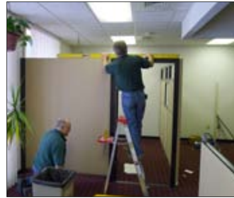
Offices were created out of the second-floor lunchroom in Building W.
