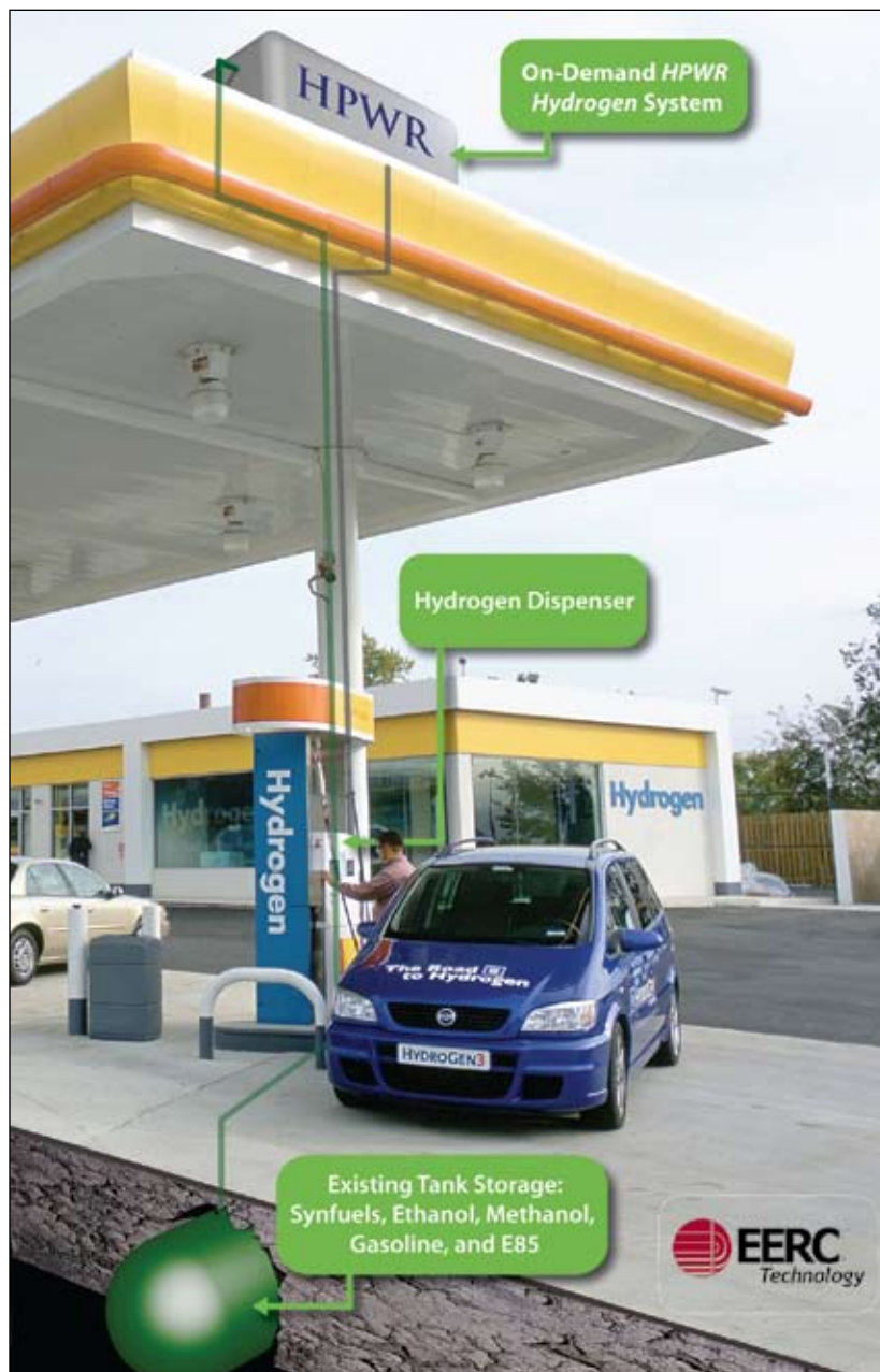
An illustration of a hydrogen-fueling station (HPWR stands for high-pressure water reforming).
