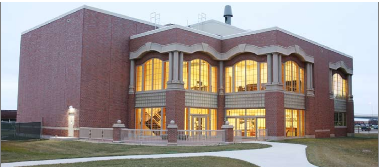
The NCHT demonstration building.
